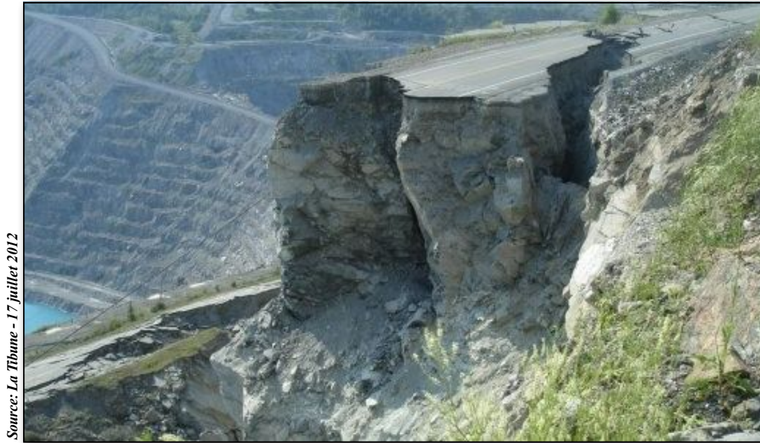
Collapse of Road 112, two sections of the road slid to the bottom of the mine in 2012.
