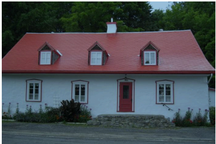
House situated at 130 Chemin Royale in Saint-Joachim
