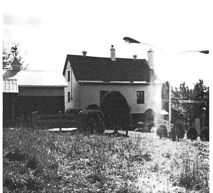
Photo d: In 1998, northside rear view
